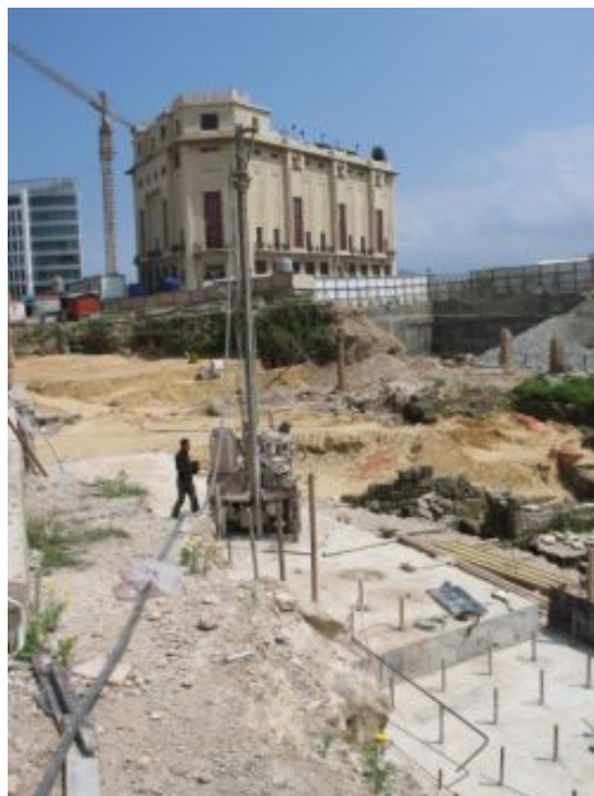
Fig. 2: The site during construction and landscaping works
